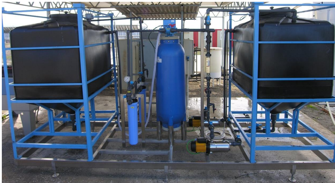
Figure III.11: UWWTP effluent pretreatment filtration system available at the PSA. Consisting out of a feed tank for UWWTP effluent, a sand filter (75 \mu\text{m} ) and two cartridge filters (25 \mu\text{m} and 5 \mu\text{m} ) in series, and a storage tank (1 \text{m}^3 ) for the filtered UWWTP effluent. The systems flow is powered by two centrifugal pumps.
